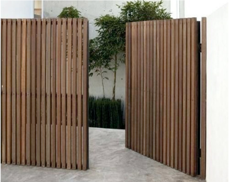
Feature Screen Fences to Road Frontage. 2x 2.5m wide x 1.5m vertical batten screen with powder coated black steel frame.
