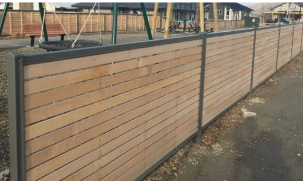
(Boundaryline Fencing or similar) 1.8m ColourSlat Signature Timber Fencing (to road frontage internal boundaries)
