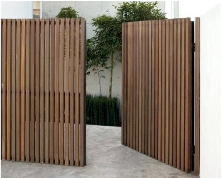
Feature Screen Fences to Road Frontage. 2x 2.5m wide x 1.5m vertical batten screen with powder coated black steel frame.
